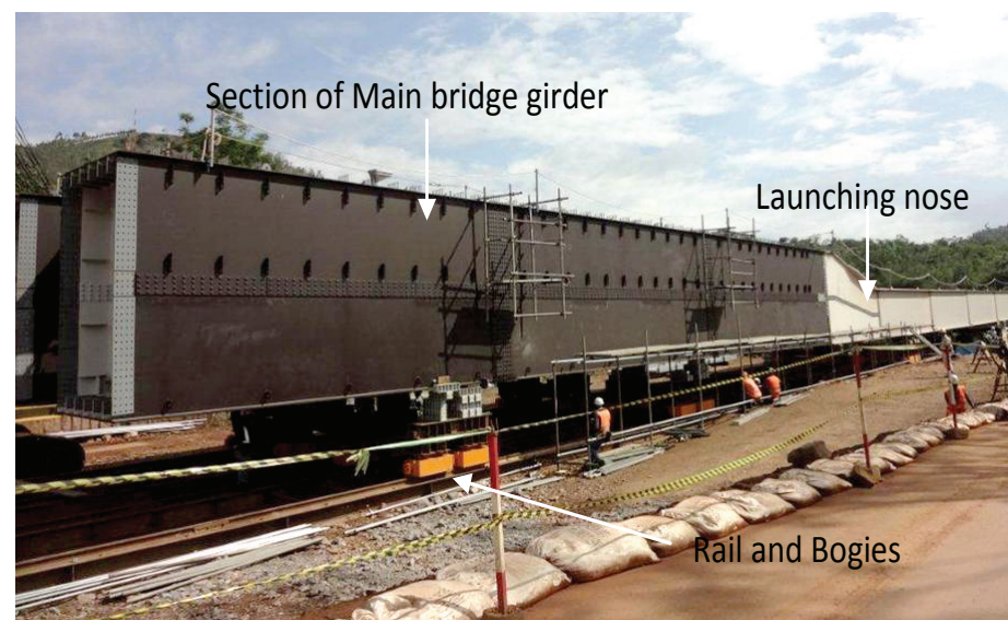
Assembled girder elements and launching nose.
